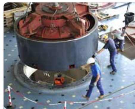
Maintenance work - A. Dumont pump station
